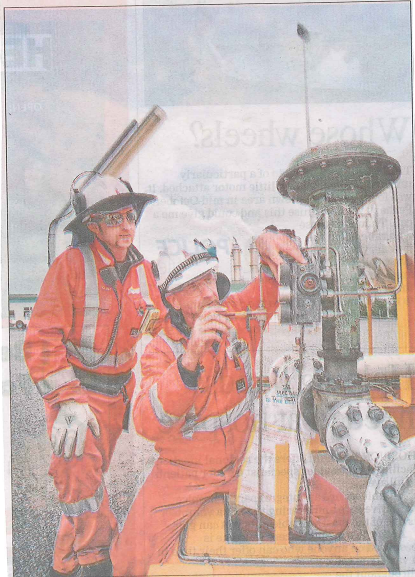
Geared up: Paul Crighton, left, maintenance technician at Shell Todd Oil Services' production station at Kapuni is assisted by area technician, Clint Hill, during a routine maintenance on process equipment at the plant. Photo: CRAIG BATES
